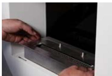
Place the burner(s) in the insert/ opening.
